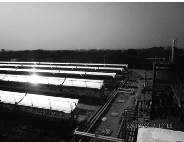
Parabolic Trough Field and the steam generation in the power plant
