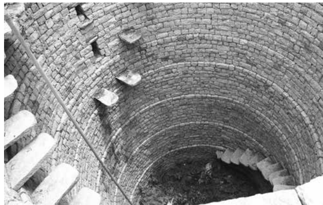
Figure 2. The open wells have dried up in most parts of peninsular India, where borewell pumping has lowered the water table drastically (Photograph by: Kirubakaran Jeremiah)
