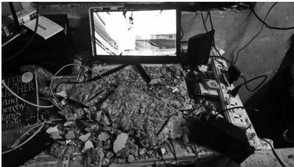
A picture of the result of the fallen ceiling debris. Courtesy Tushar Singh Thakur.
